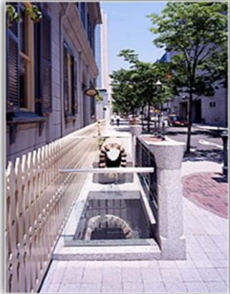
Storm sewer made of Brick (Legacy of Urban Works)
